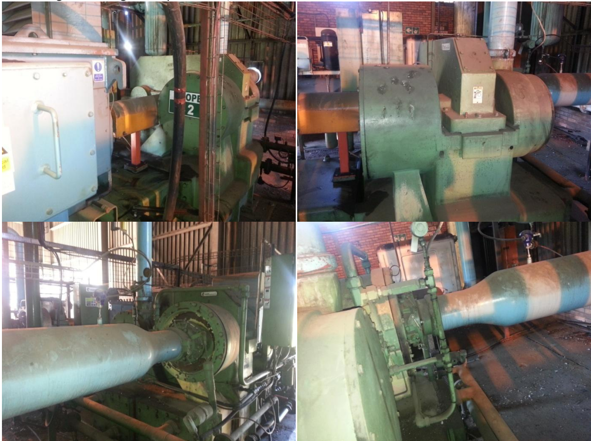
Figure 1 - Centrifugal Multistage Compressor
