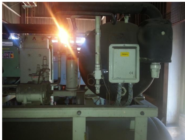
Figure 5 - Air Dryer and Cooling System
