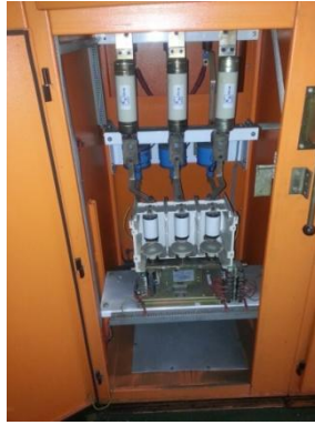
Figure 10 - Electrical Breaker and Switchgear
