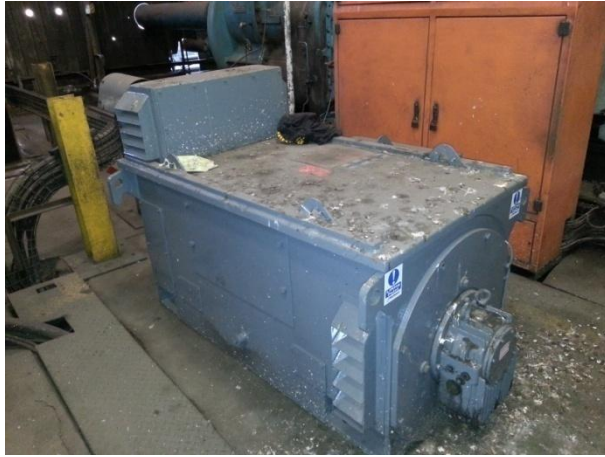
Figure 12 – Spare Compressor Motor
